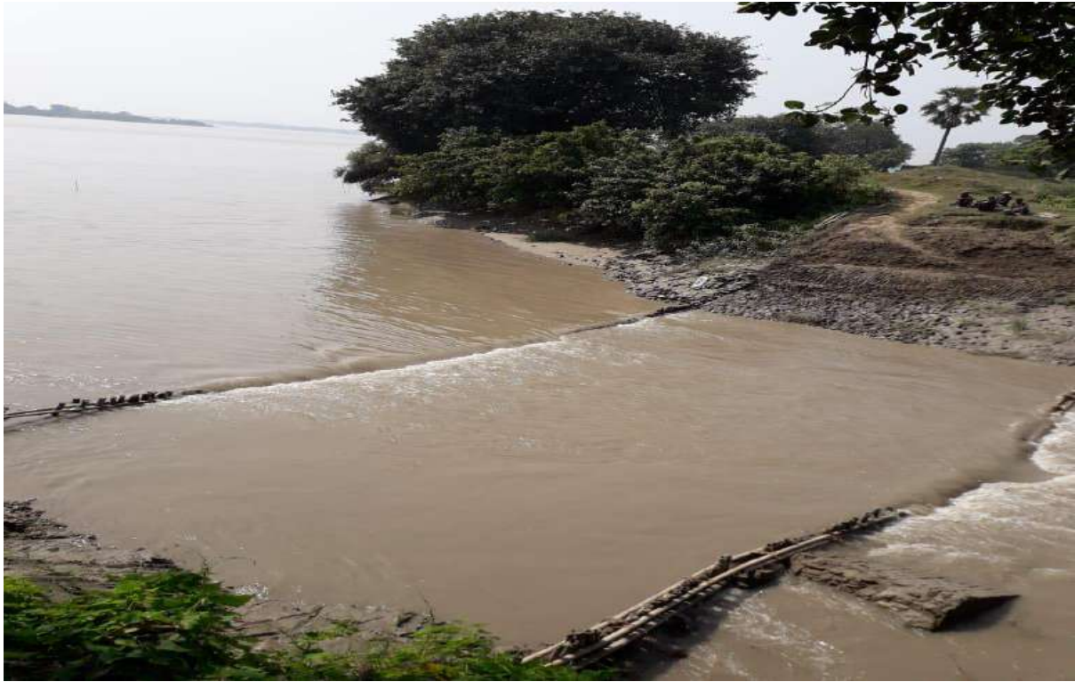
Silt Rich Water Entering Silt-Tanks
